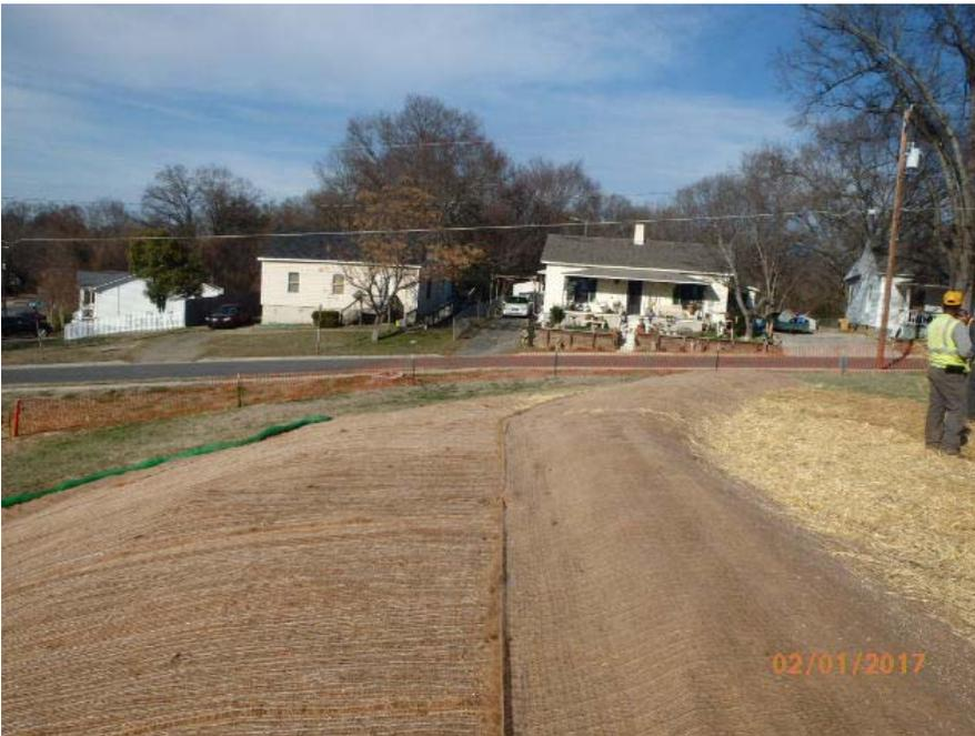
**Photo 4.** Completed construction of interim embankment stabilization on-site.
