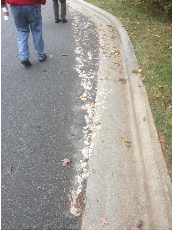
**Photo 1.** Asbestos released into the street due to erosion of on-site embankment.
